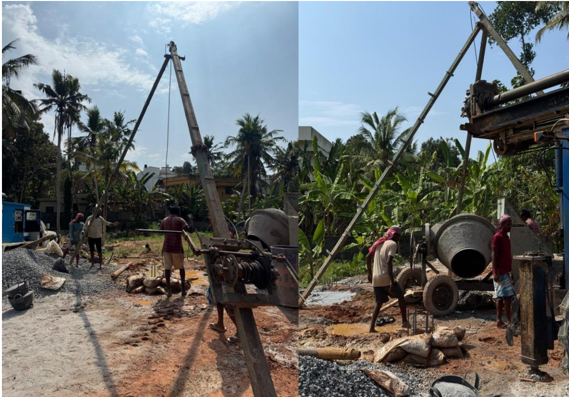
Site Visit on Pile Foundation Construction in a Waterlogged Area
