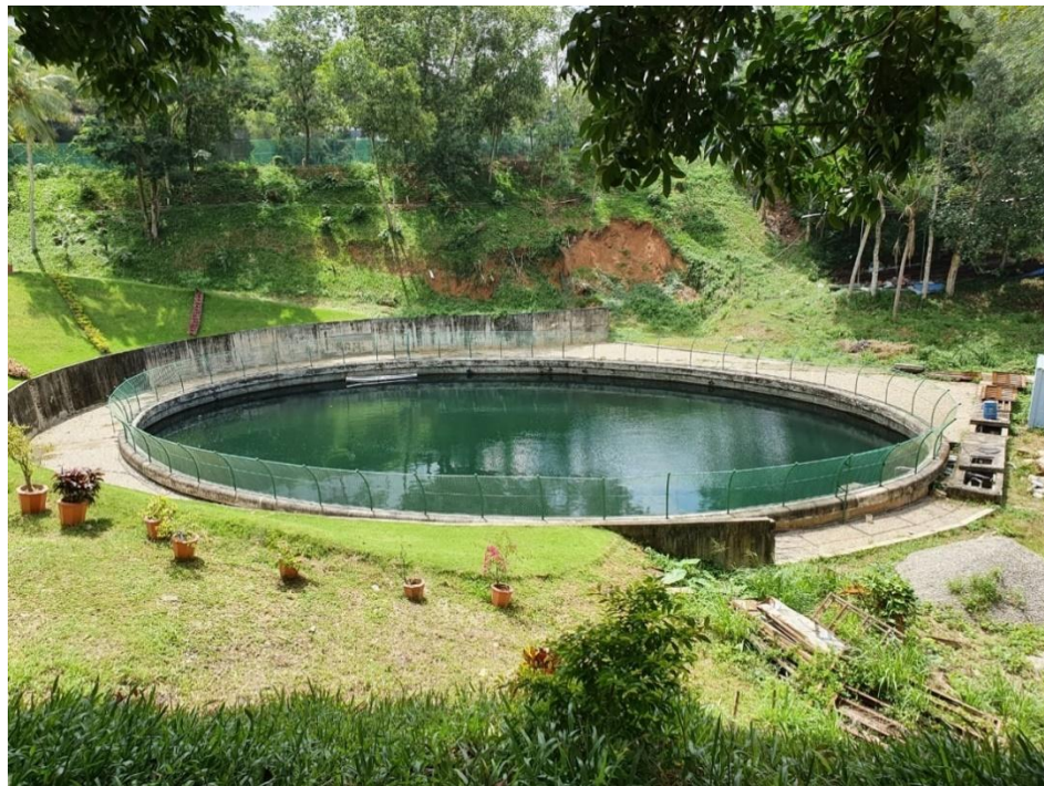
Fig. 2 Elliptical shape reservoir of rainwater harvesting system
