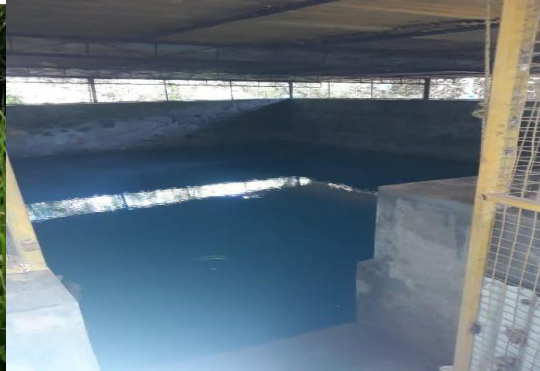
Fig.4: Open well at Mar Aprem Hostel
