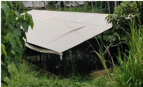
Fig:3 Open well at Sarvodaya Vidyalaya
