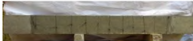
Fig 5. Ferrocement mesh wrapped beam
