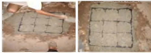
Fig.7 Construction of CFC overlay
