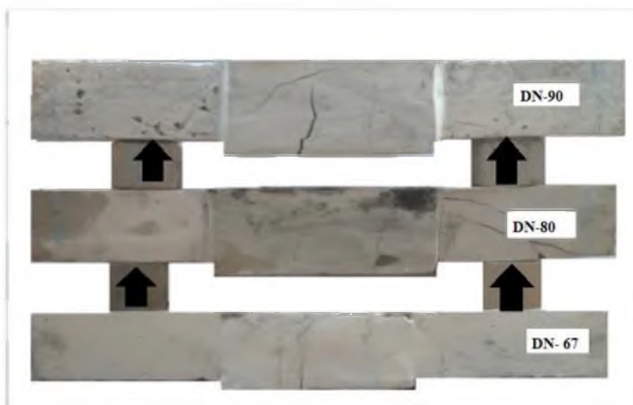
Fig. 3 Crack patterns of the retrofitted beam specimens.
