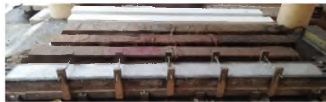
Fig.3 Beams kept for curing
