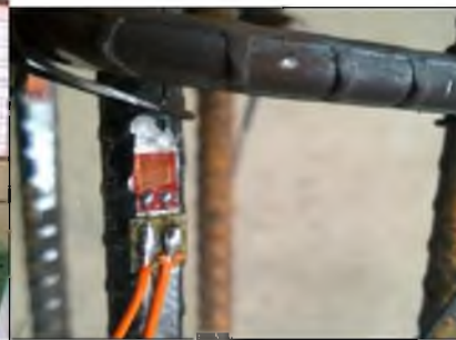
Fig 5. Connection of strain gauge
