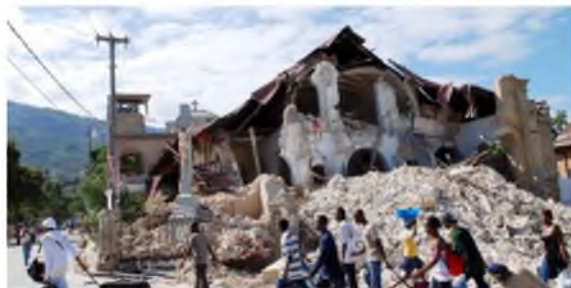
Fig.1. Failure of an URM building during 2010 Haiti earthquake [1]
