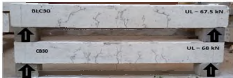
Fig 3. Crack pattern of CB30 and BLC30 beams
