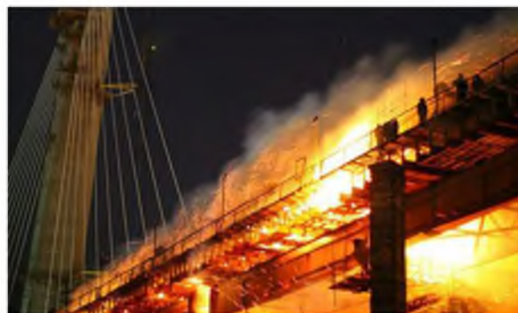
Fig.1 Bridge constructed over Zolotoi Rog Bay caught fire, Vladivostok
