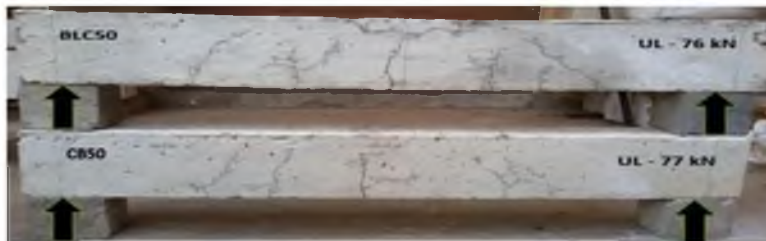
Fig 4. Crack pattern of CB50 and BLC50 beams
