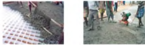
Fig.4 Cell filled pavement under construction and compaction of concrete [6]
