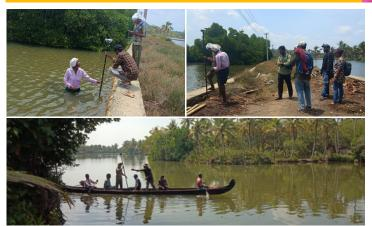
Topographical Survey as part of the construction of Arinalloor Peringalam Bridge. Kollam was conducted by the Dept. of CE, for Kerala PWD
