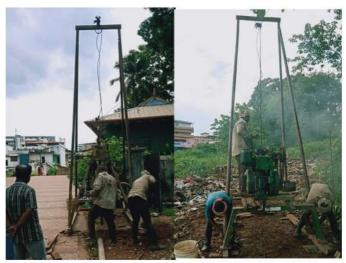
Soil investigation works were done for Minor Bridge Construction at Kottarakkara (PWD) and Sewerage Treatment Plant construction at Karunagappally, Pathanamthitta, and Nedumangad (KWA).
