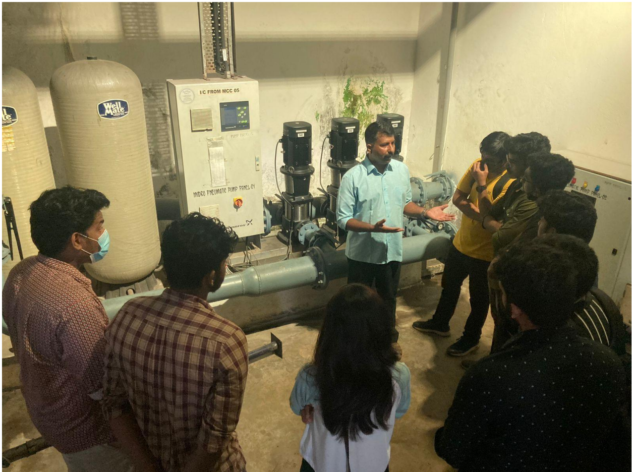
Fig ( 1 ) Mr .Noushad explaining hydro- pneumatic pump
