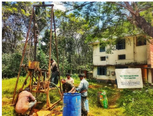
Photo#8: Soil investigation work at Government V H S S Keezhvaipur
