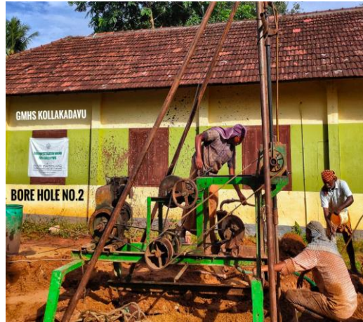
Photo # 4 : Soil investigation work at Government Muhammadin High School at Kollakadavu
