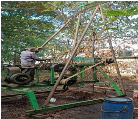
Photo # 1: Soil investigation work at Killipalam
