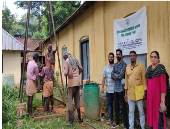
Photo # 3 : Soil investigation work at Educational complex at DIET, Kottarakkara
