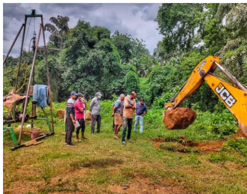
Photo#6: Soil investigation work at Government ITI Ranni
