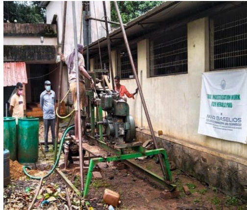
Photo # 5 : Soil investigation work at Thiruvalla Hospital
