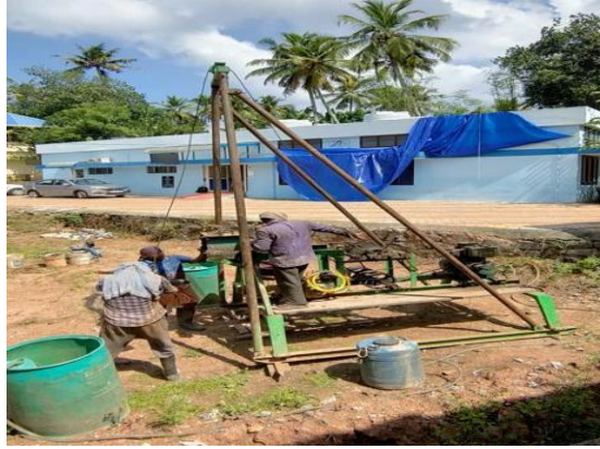
Photo # 2 : Soil investigation work at Taluk Hospital, Santhivila
