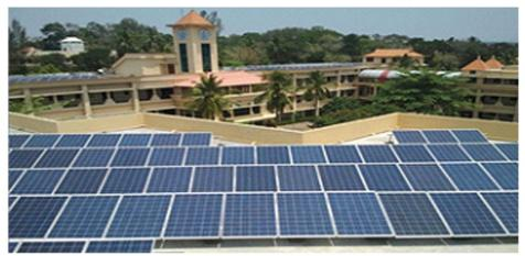
The first Solar Power Plant with a capacity of 100 kWp was commissioned in April 2013, and the second one of 100 kWp in August 2018. The total project outlay was approximately Rs.267.00 Lakhs. Currently, the power is fed to the grid during off-load times and holidays. It is observed that the Utility's bill amount is remaining without much increase in spite of the increased usage of electricity on the campus. The significance of the venture can
